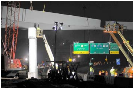
Setting girders for Exchange Avenue Bridge on April 7 th . Photo: stltoday.com
