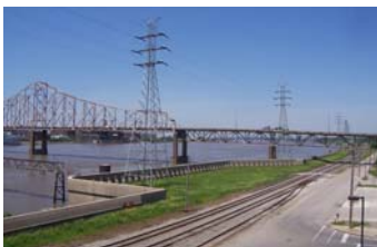
Metro East Sanitary District (MESD) flood wall in East St. Louis. Photo: MESD
