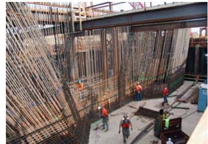
Installing tower steel. Photo: MoDOT
