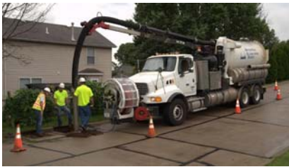
Stormwater maintenance. Photo: MSD
