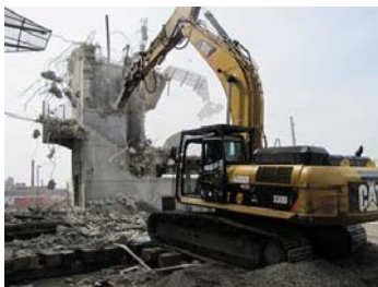
Demolition at Grand Avenue MetroLink station. Photo: Metro
